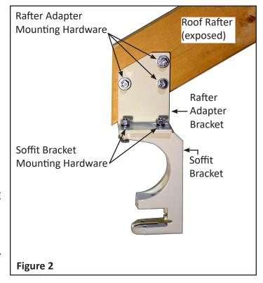
3. Refer to the **Owner's Manual & Installation Instruction (Appendix C – Soffit Mount)** to locate the rafters in the areas in which the **Rafter Adapter Brackets** must be installed.
